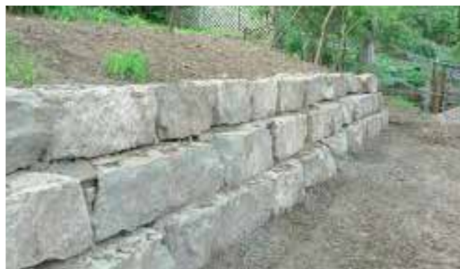
Figure 2: Armourstone on site and in place for decorative use
