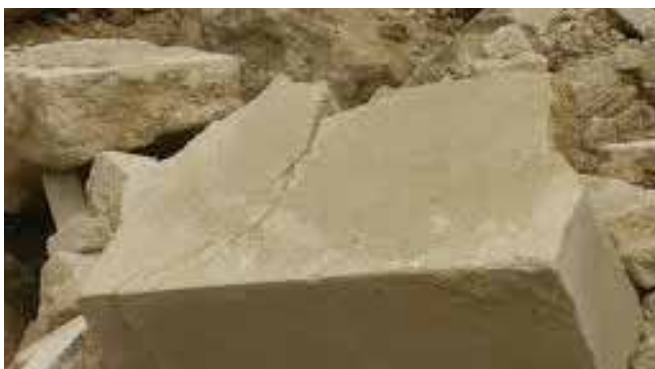
Figure 5: Cracking and defects that can affect the integrity of a structure and test results
